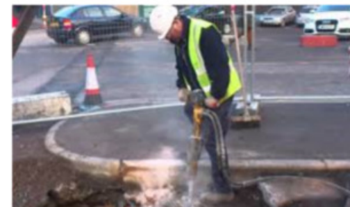
Water main break Jack hammering
