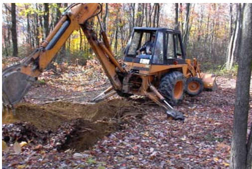
Test pits being dug for soil evaluation.
